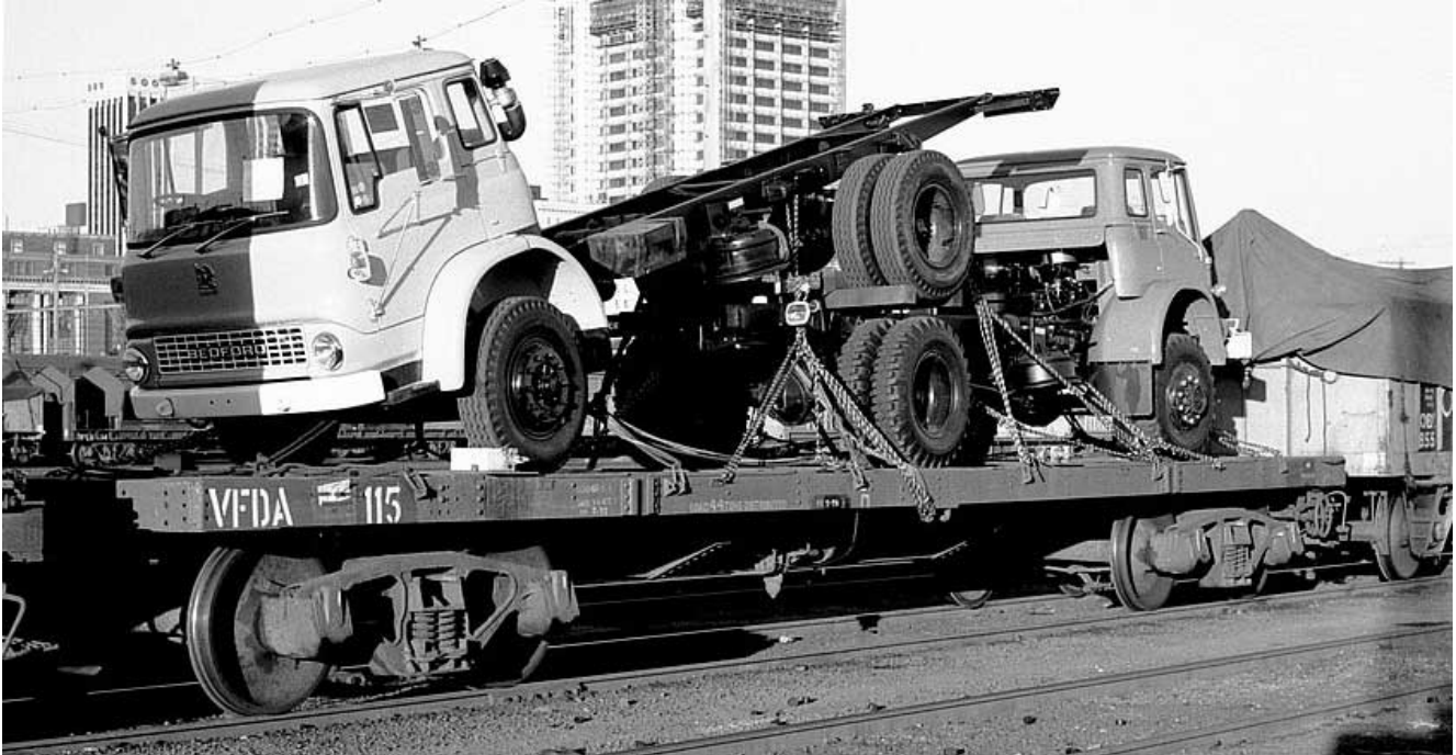
VFDA 115 fully loaded Centre Yard Melbourne 14/07/1979. Photo courtesy of Rob O'Regan.
